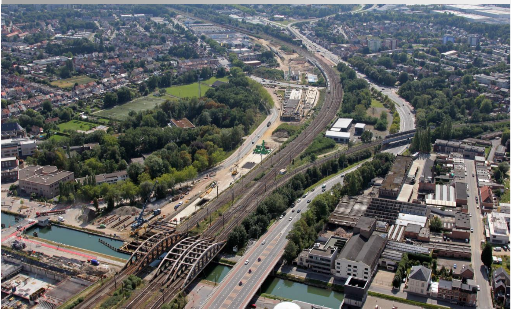
Belgium – Construction of the Railway Bypass in Mechelen
