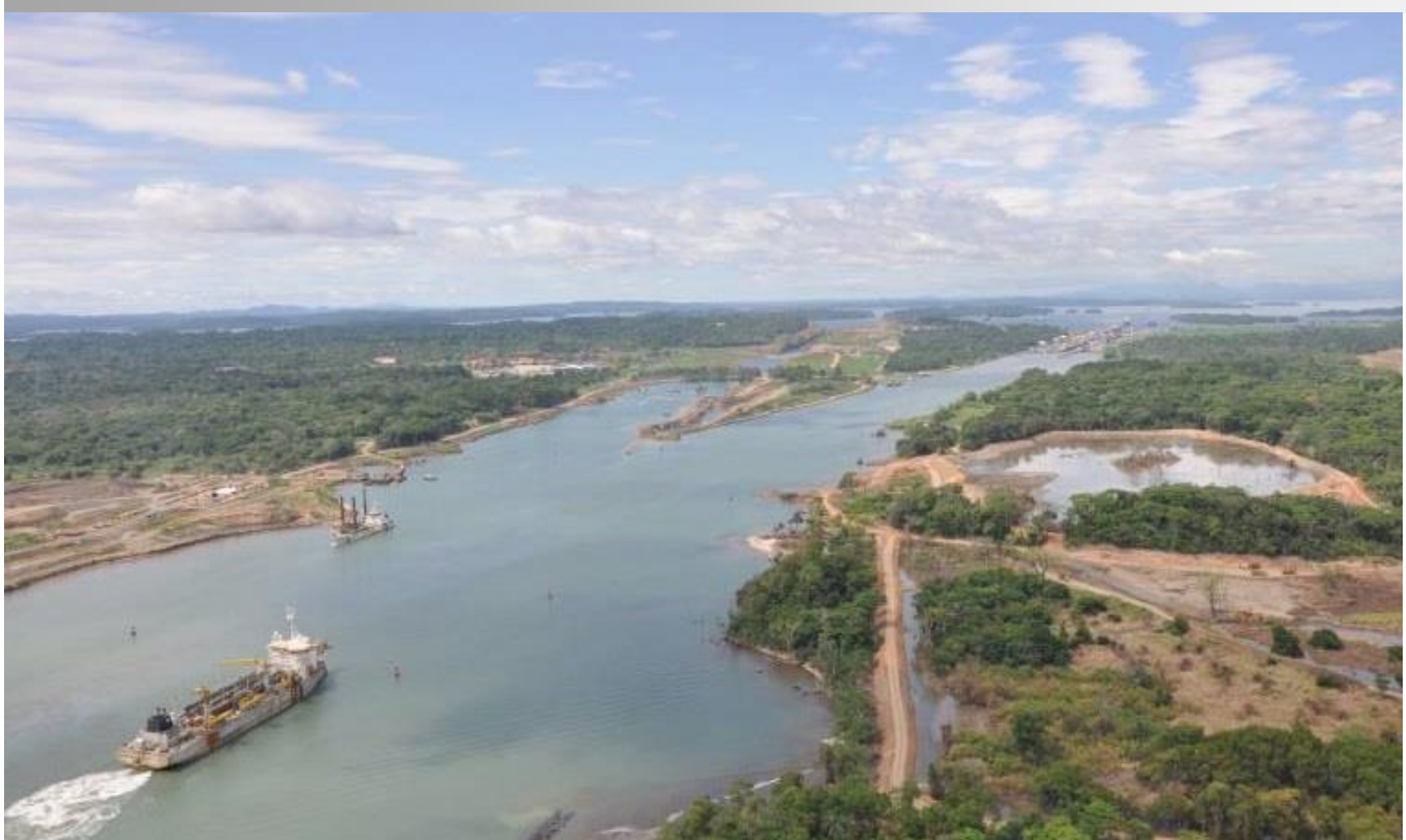
Panama Canal - Widening and Deepening of the Atlantic entrance & North Approach Channel to the Third Set of Locks
