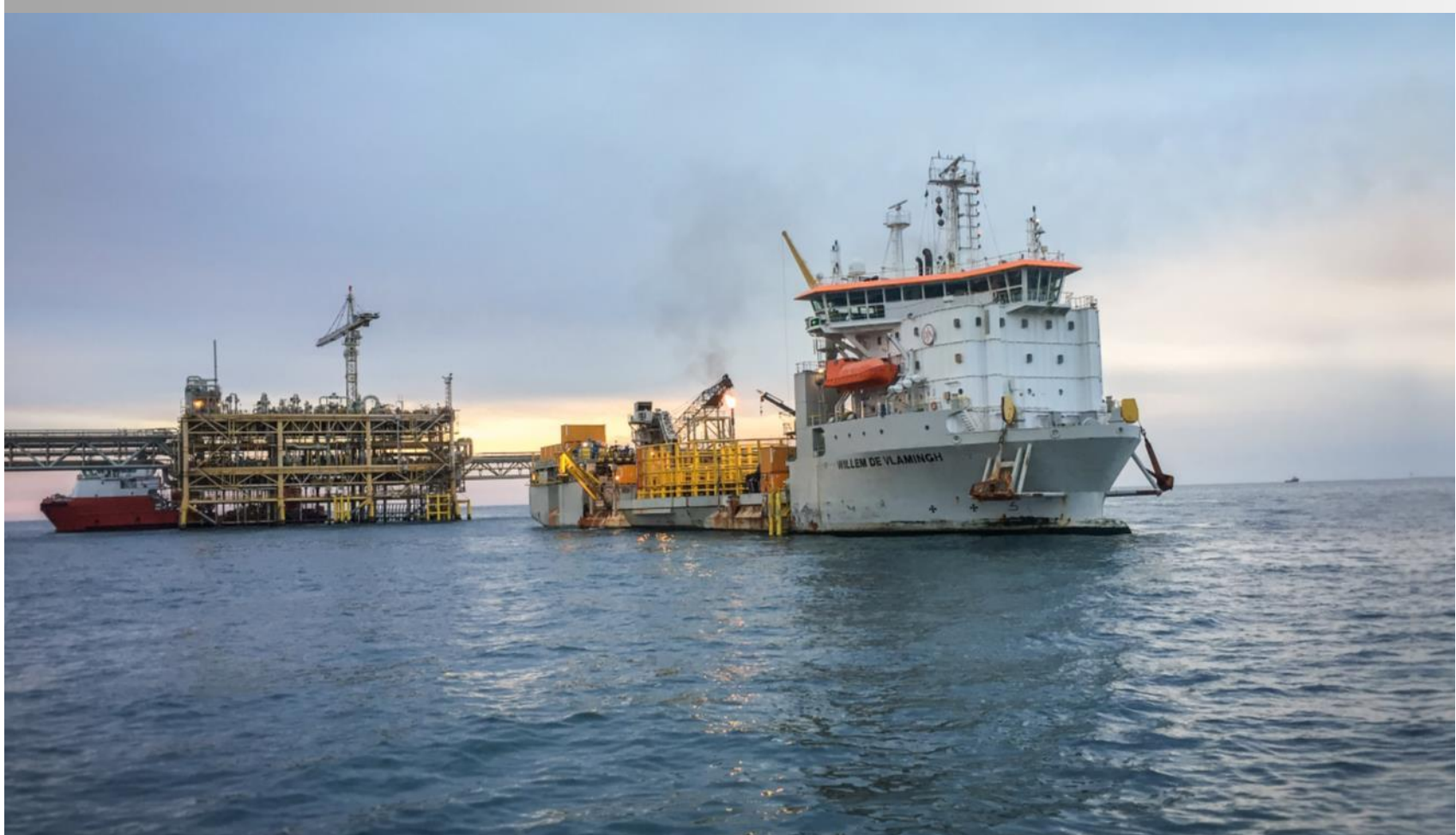
Saudi Arabia – Transport and Installation of Subsea Power Cables for the Marjan Zuluf Field Facilities - CLV Willem de Vlamingh
