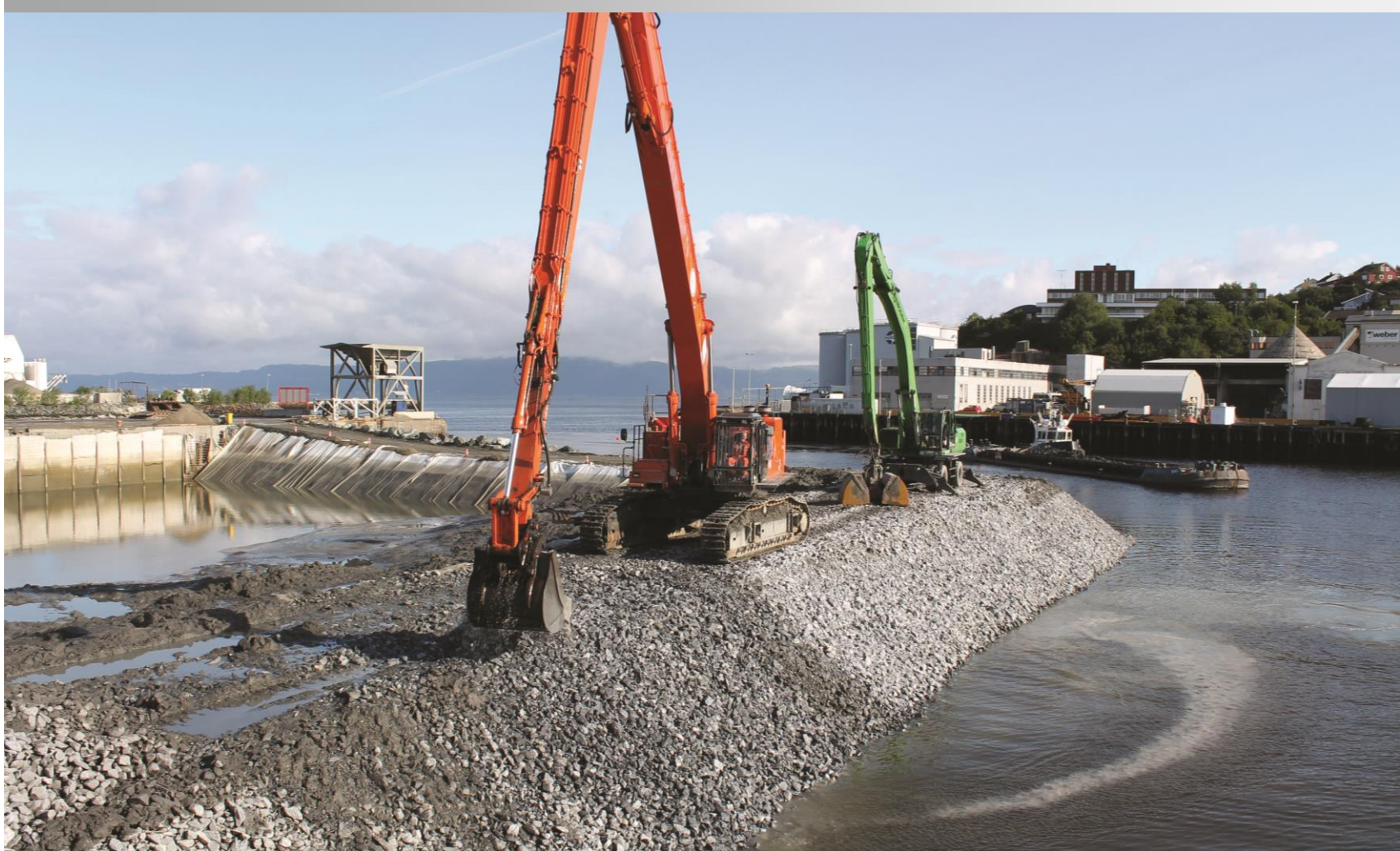
Norway – Dredging and Revalorisation of Contaminated Sediments for Land Expansion in the Port of Trondheim
