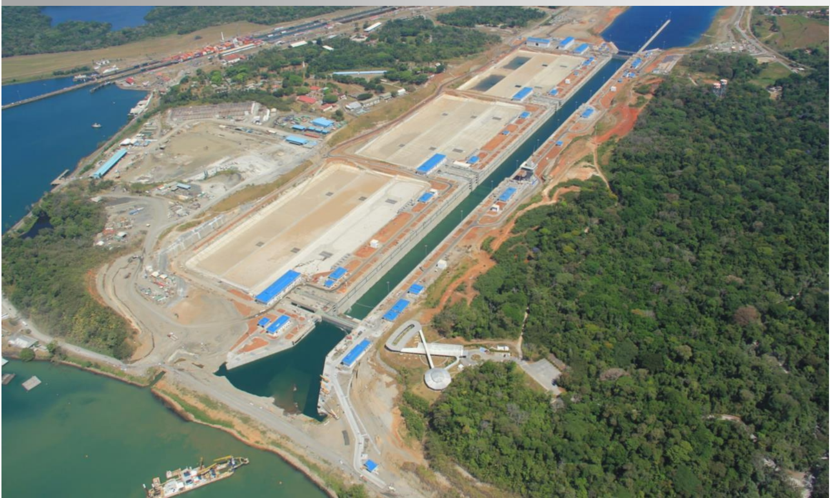
Panama – Design and Construction of the Third Set of Locks of the Panama Canal
