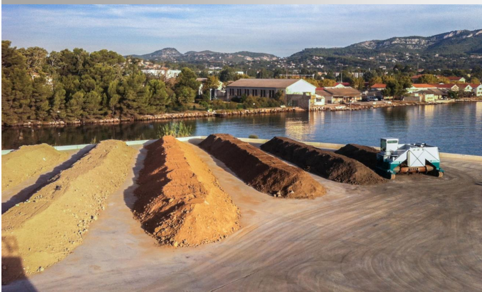
France - Construction and Operation of a Groundwater and Sediment Treatment Centre in La Seyne-sur-Mer
