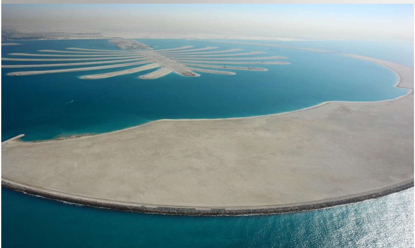
UAE – Palm Island II (Jebel Ali) in Dubai Reclamation and Stone Revetment Works
