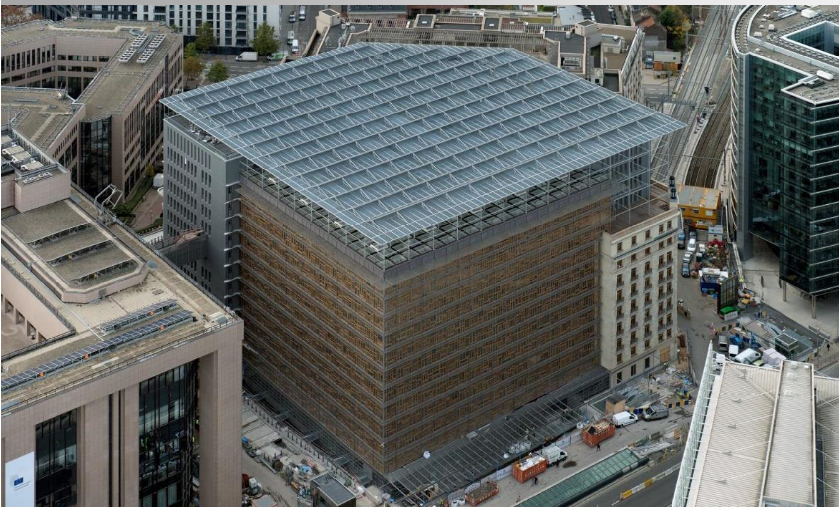
Belgium – Construction of the Future European Council seat ‘Résidence Palace’ in Brussels
