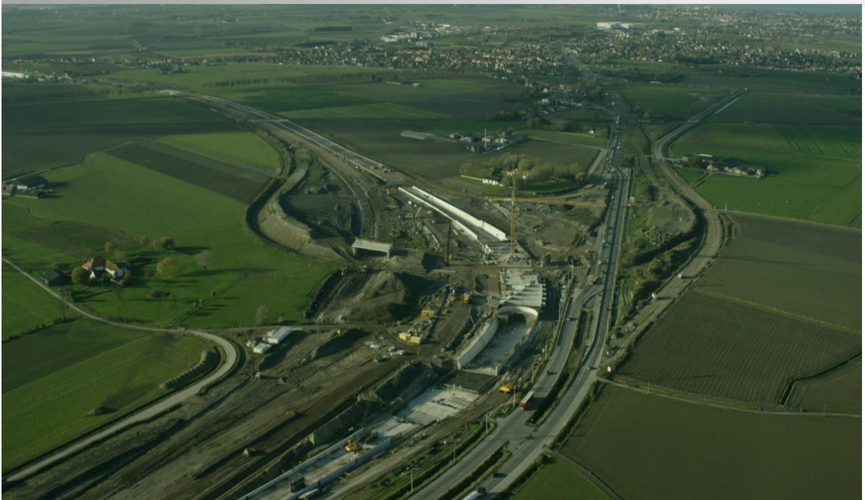
Belgium – Construction of the Highway Connection A11 Bruges-Westkapelle
