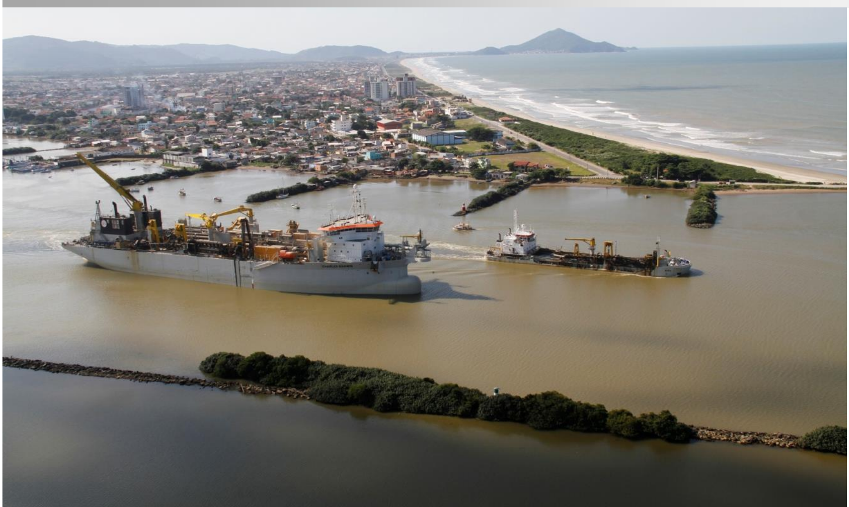
Brazil – Access Channel and Port Basin Dredging in Itajaí TSHDs Charles Darwin and Niña
