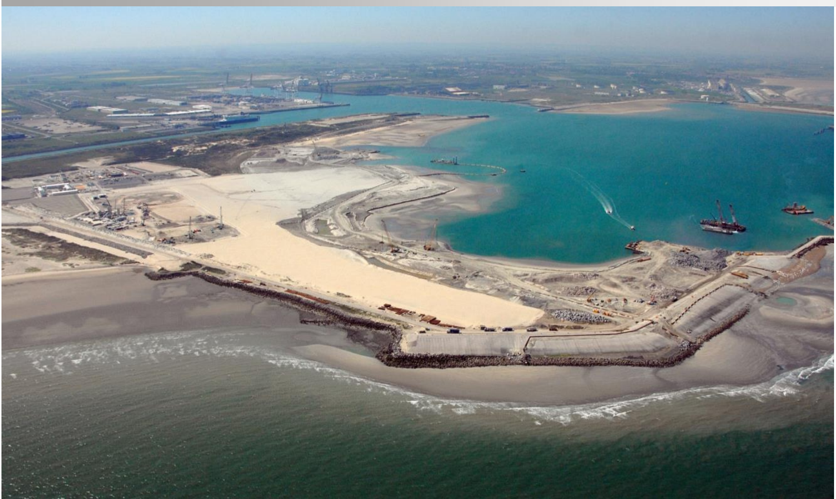
France - Construction of Harbour Facilities for the Future LNG terminal in the Outer Harbour of West-Dunkirk
