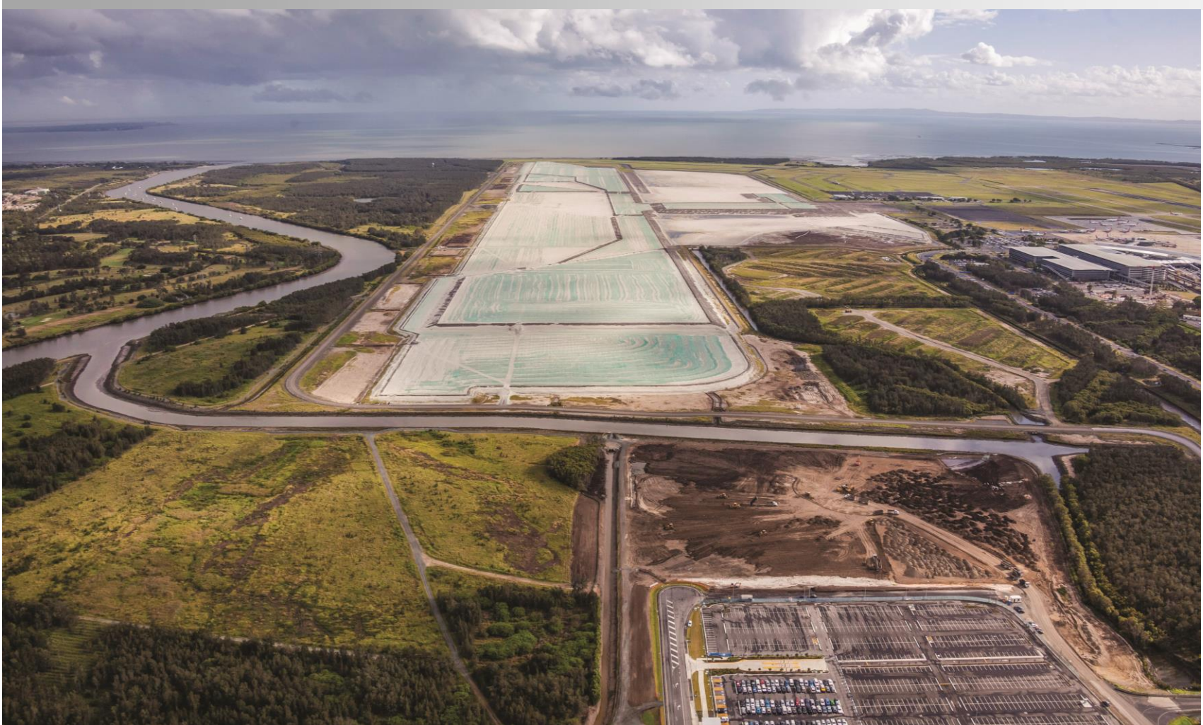
Australia – Land Reclamation Project for the Construction of a New Parallel Runway at Brisbane airport
