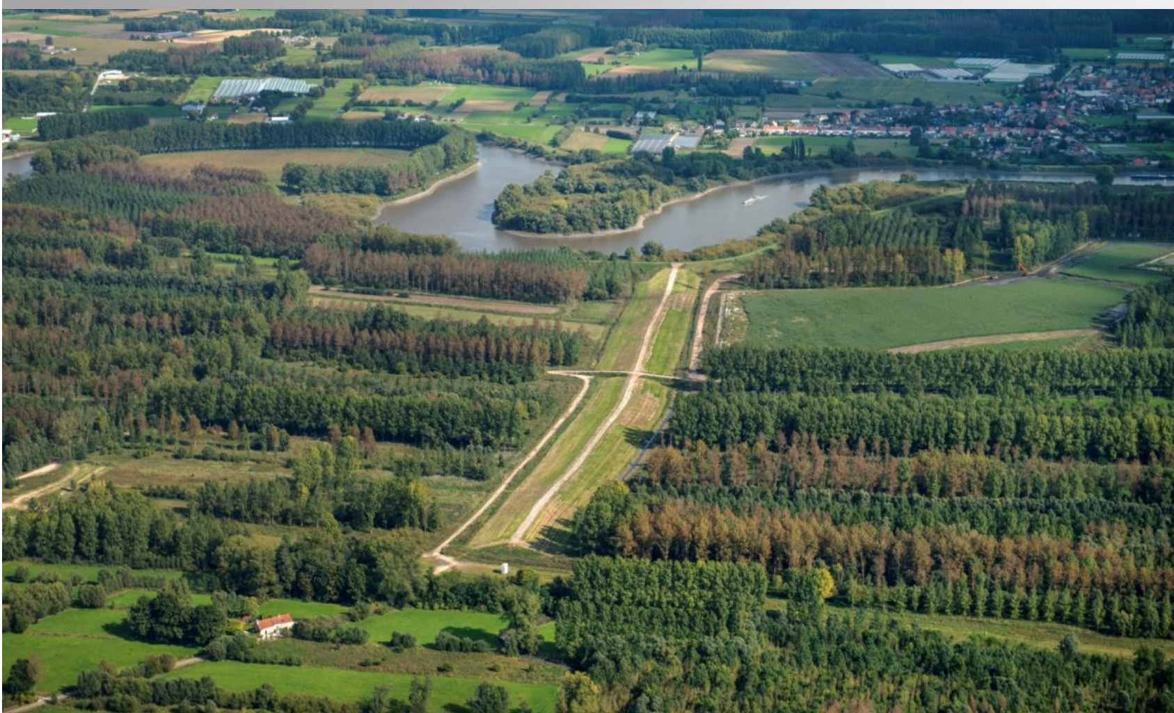
Belgium - Construction of a Ring Dike in Vlassenbroek using Sediments Dredged in the Scheldt between Gentbrugge and Melle
