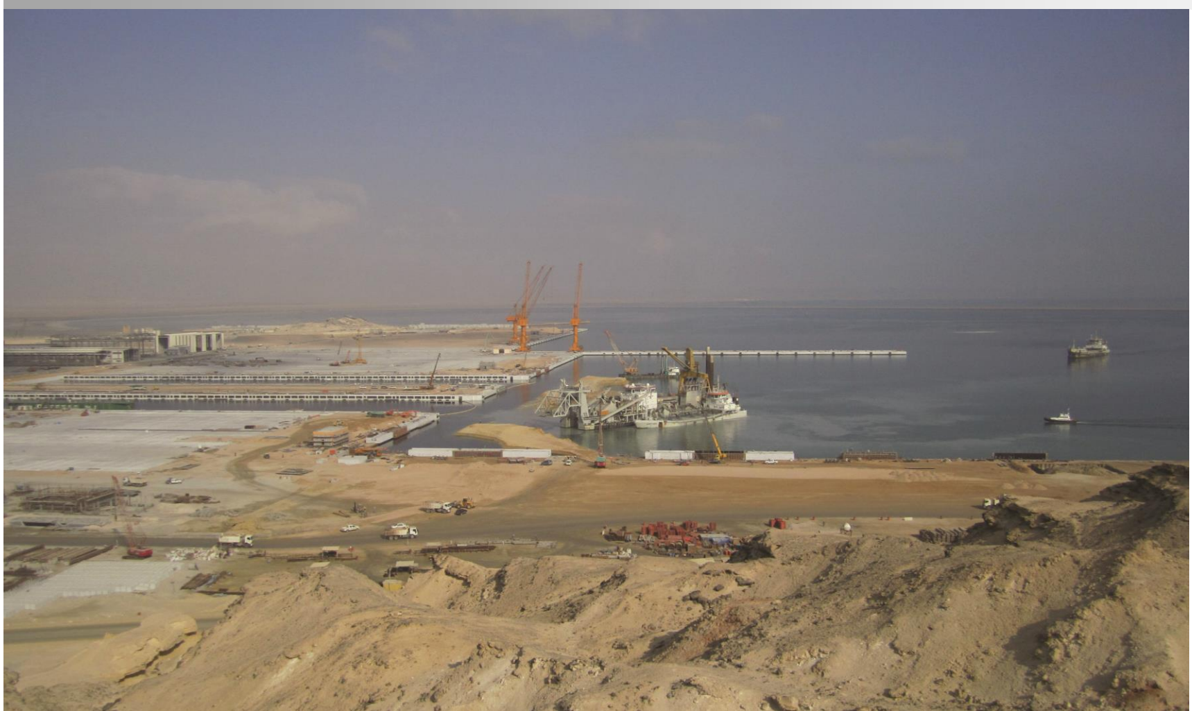
Oman – Construction of New Port of Duqm CSD J.F.J. De Nul and SHB Santiago
