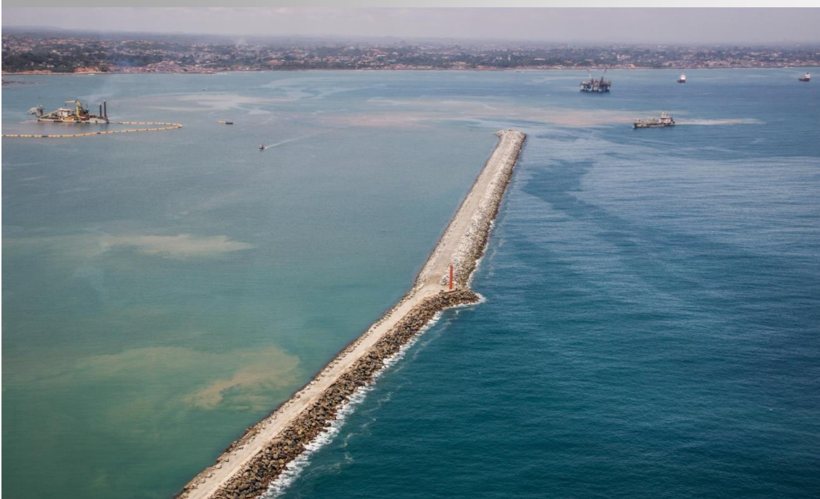
Ghana – Extension of Existing Port Infrastructure in Takoradi CSD Niccolò Macchiavelli
