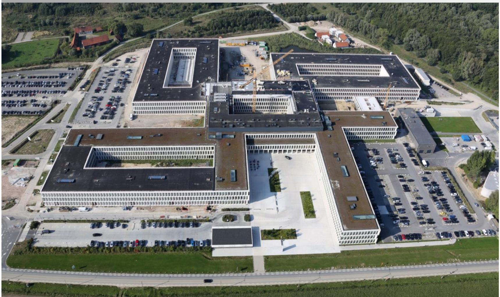
Belgium – Construction of a New Hospital in Kortrijk
