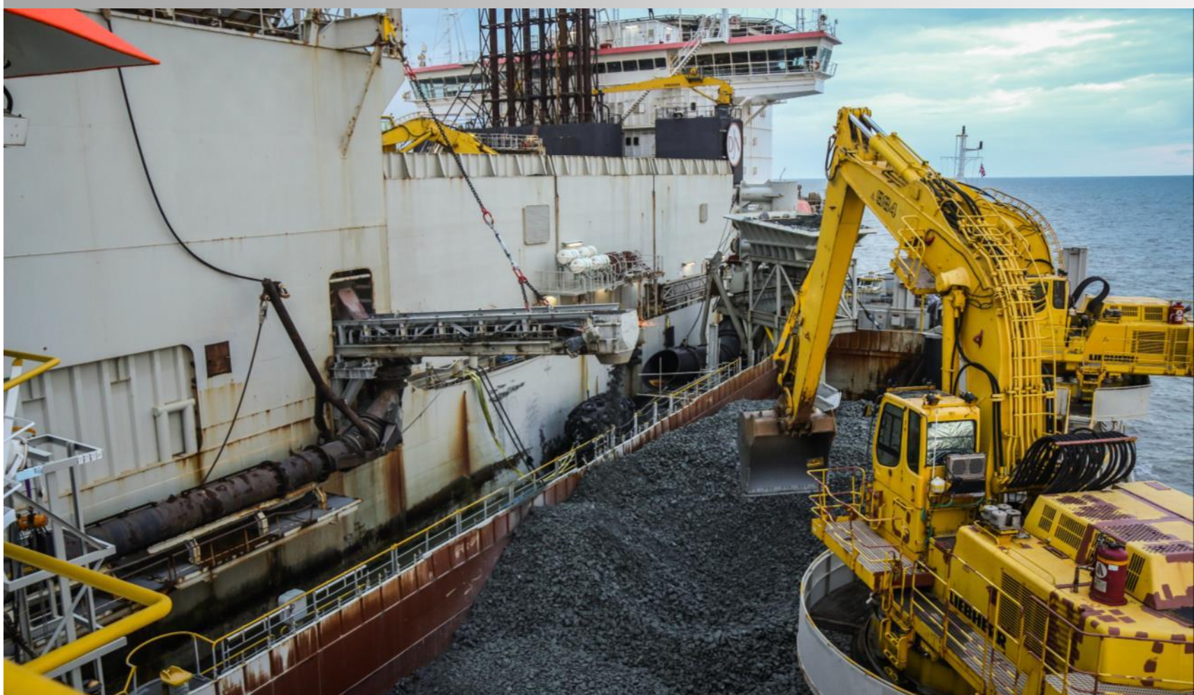
Great Britain - Rock installation Works to Protect the Foundations of the Offshore Wind Farm Gunfleet Sands – SRIV Simon Stevin & FPV Tiger
