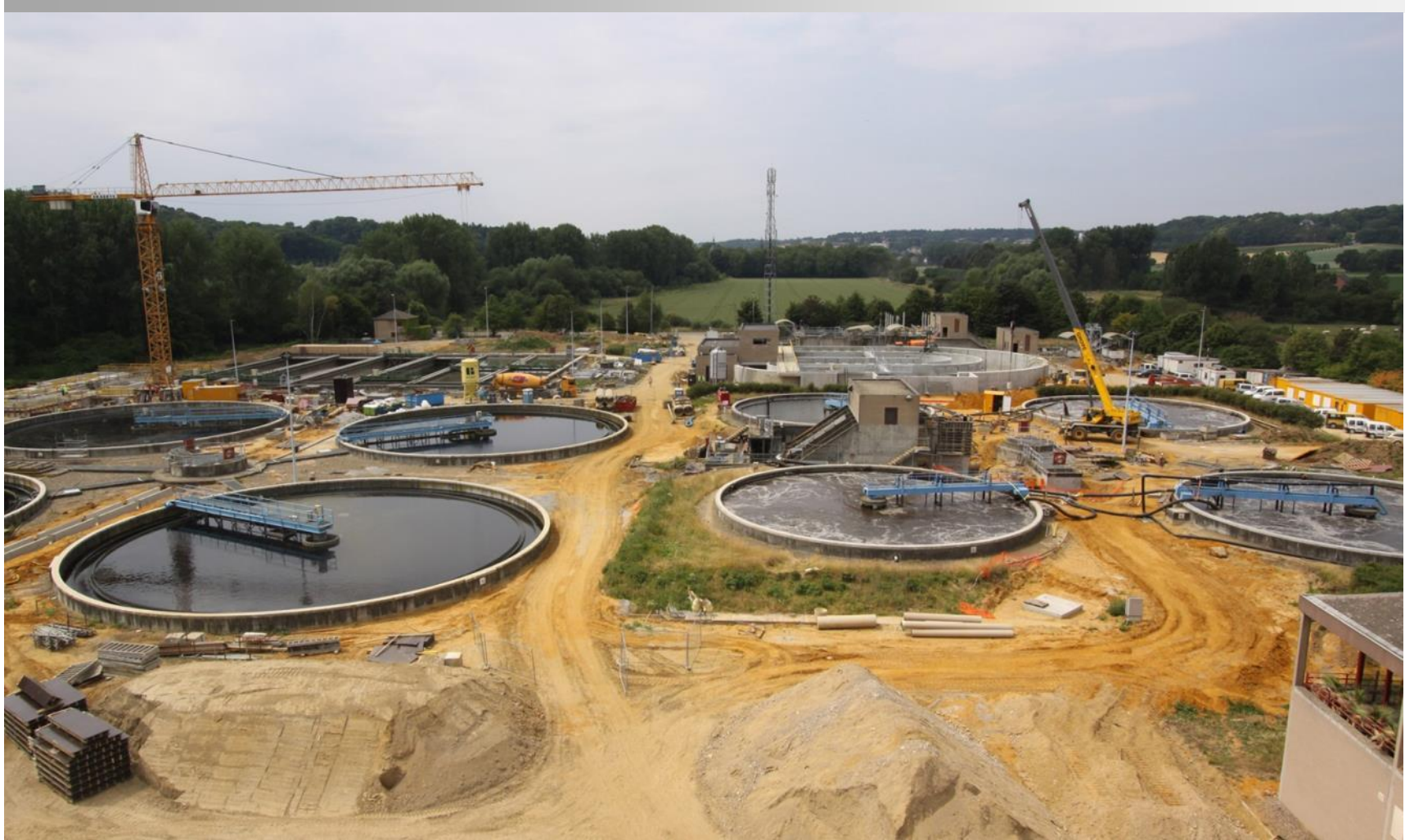
Belgium – Construction of a Water Purification Plant in Waver
