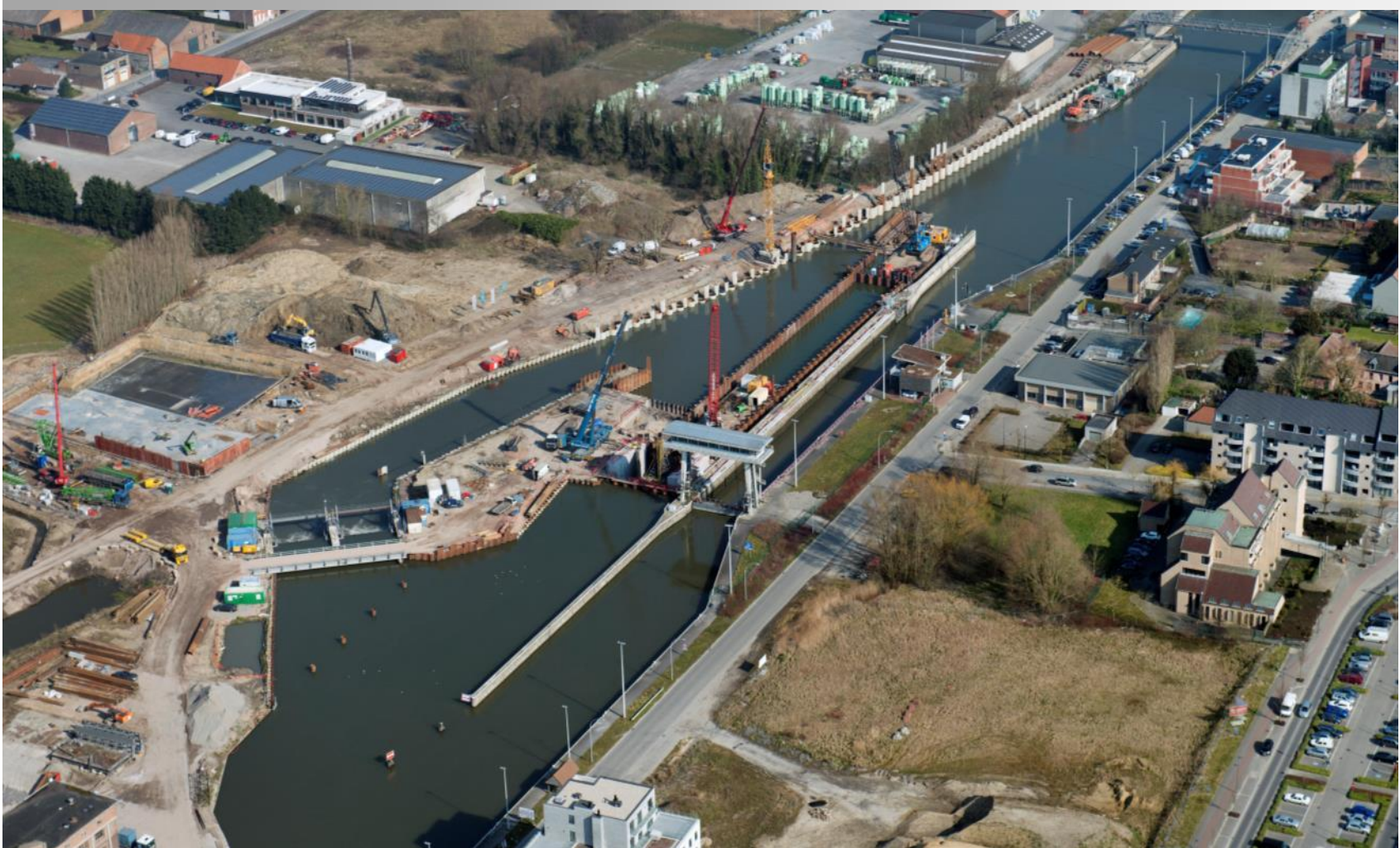
Belgium – Construction of the New Lock in Harelbeke
