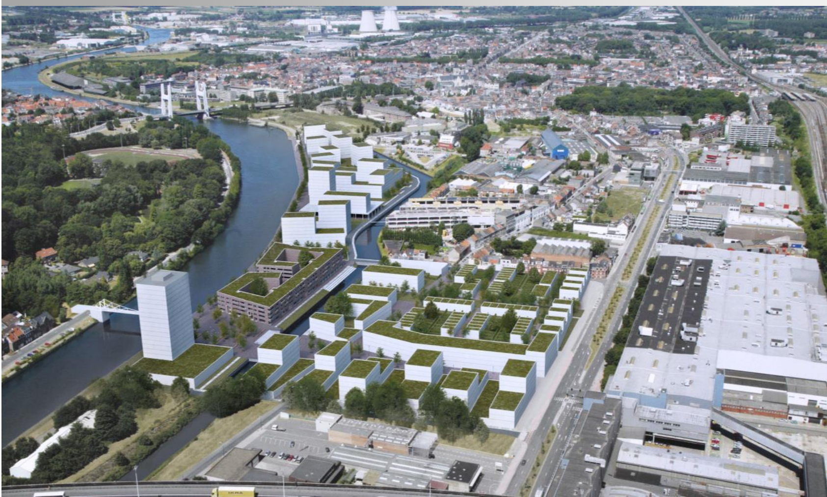
Belgium – Brownfield Remediation and Urban Redevelopment Project '4 Fonteinen' in Vilvoorde
