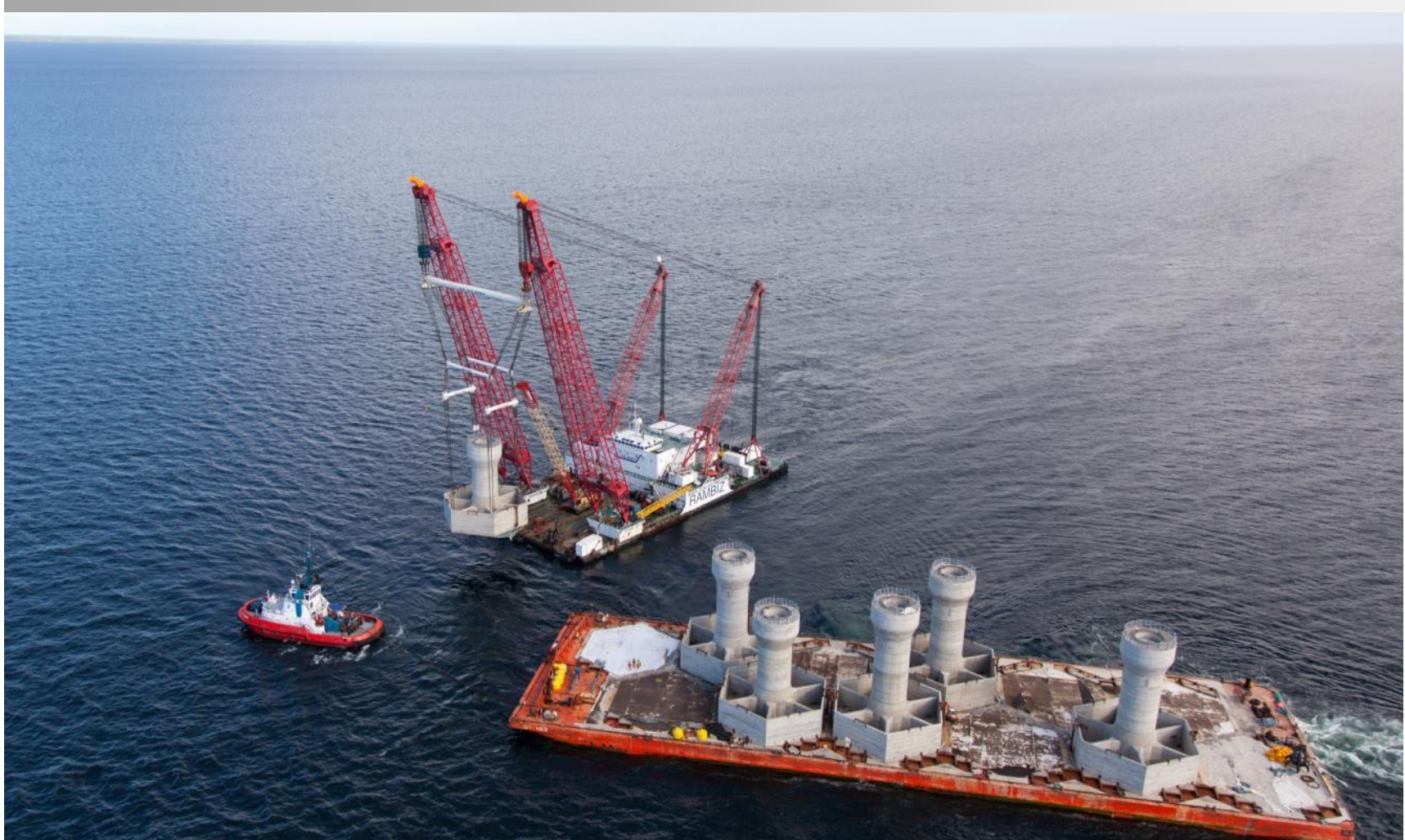
Sweden – Design, Construction and Installation of 16 Concrete Foundations for the Offshore Kårehamn Wind Farm
