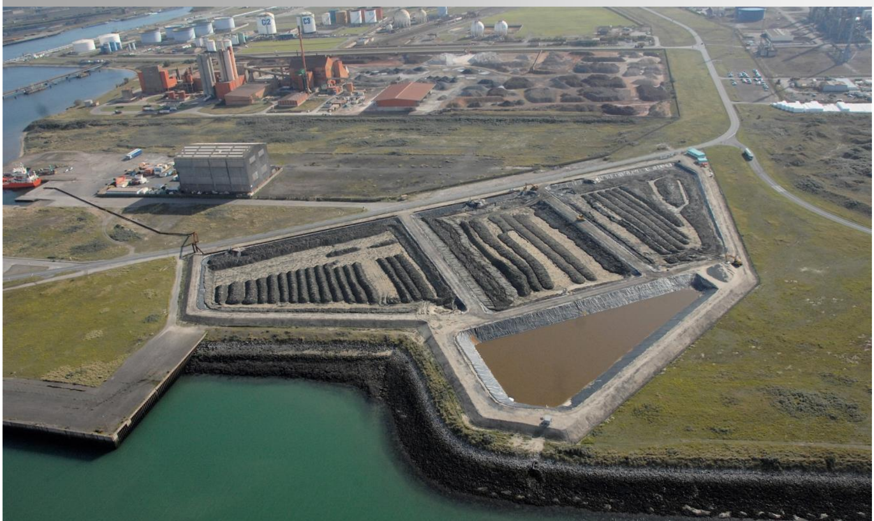
France – Dredging and Treatment of Contaminated Sediments in the Port of Dunkerque
