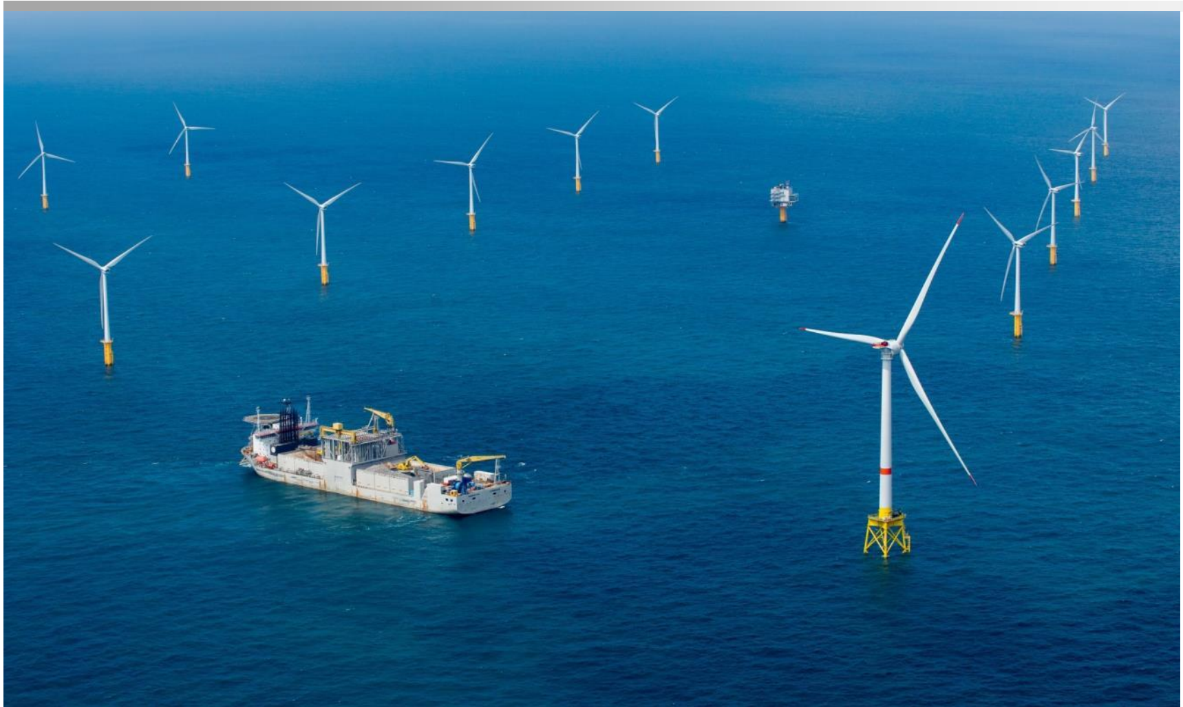
Belgium – Alstom Belwind Demonstration Project CLV Simon Stevin
