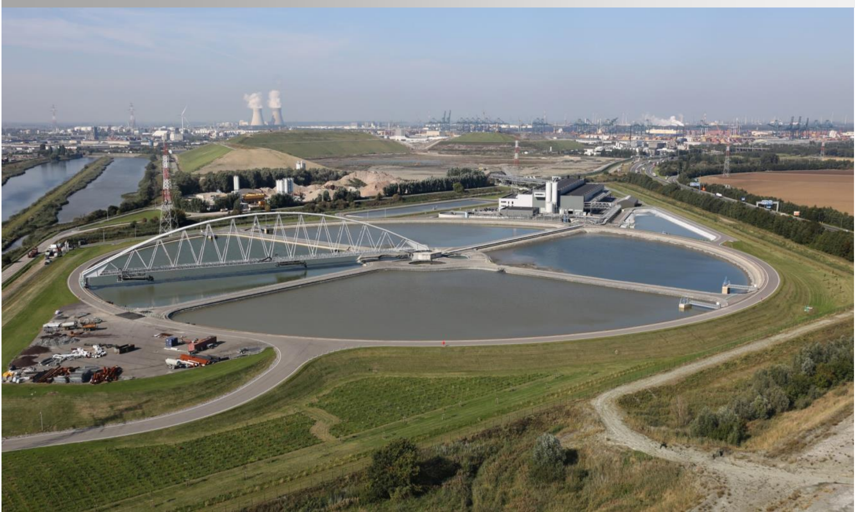
Belgium – AMORAS Project in the Port of Antwerp Mechanical Dewatering, Recycling and Application of Silt
