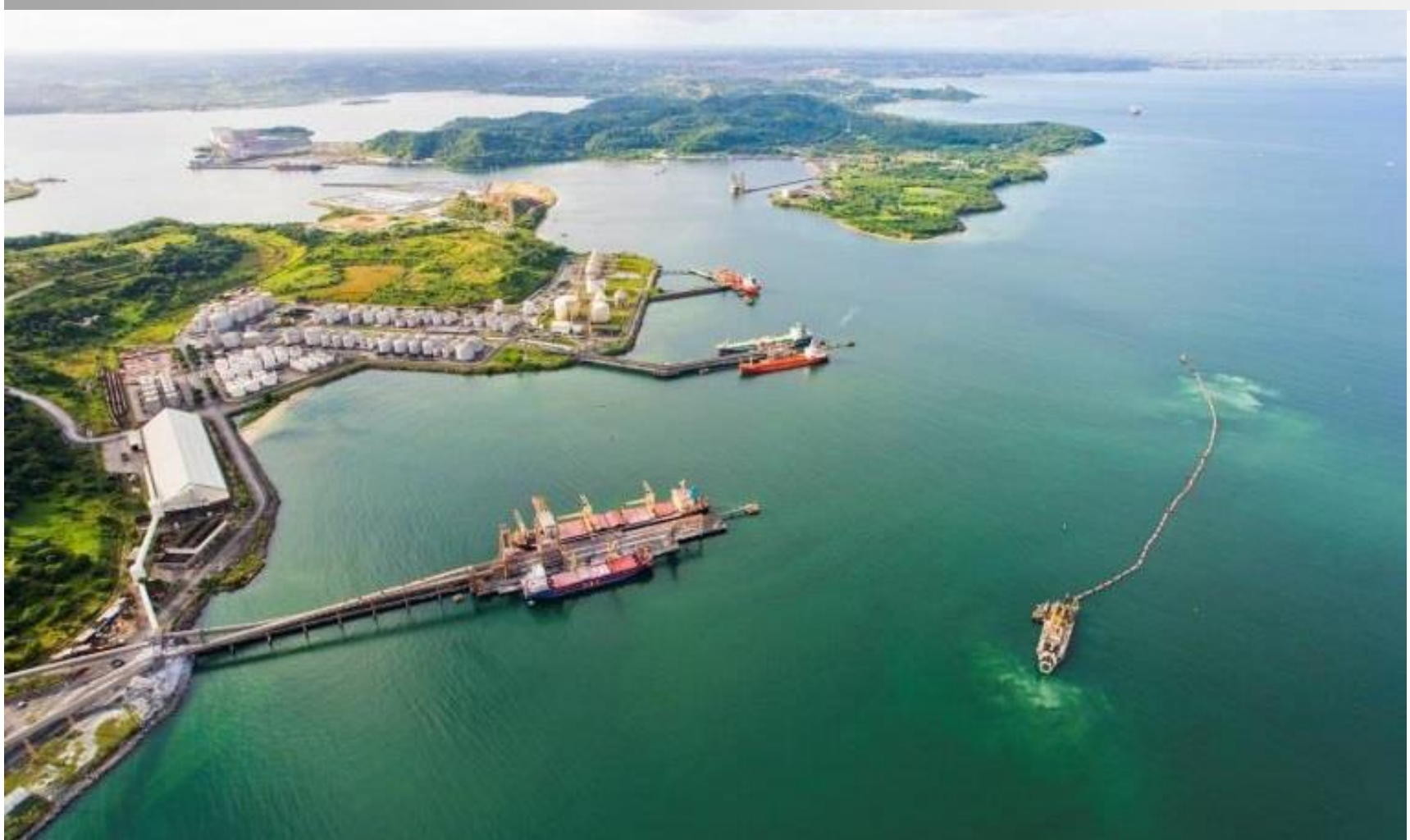
Brazil – Deepening dredging in the Ports of Salvador and Aratu CSD Hondius
