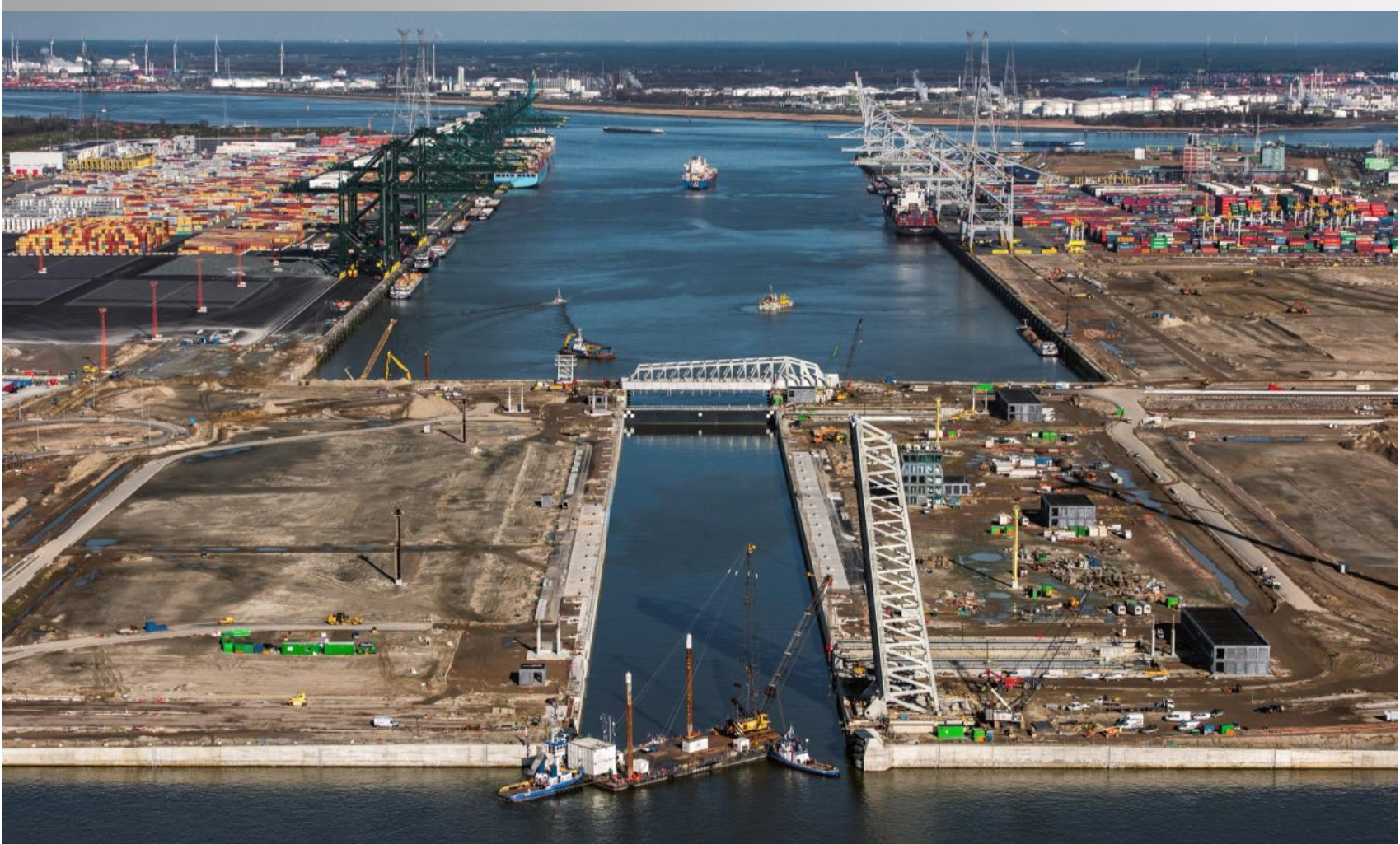
Belgium – Construction of the Deurganckdok Lock in the Port of Antwerp
